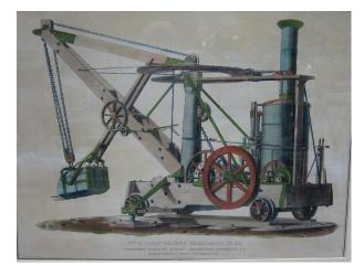
This picture was taken in 1841 and shows the earliest depiction of a type of excavator. This invention, although revolutionary for the time, had multiple drawbacks in the way it was able to operate. Firstly, it was only able to run in train track meaning that when it was used temporary tracks were placed at the time that
